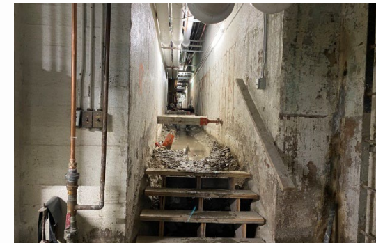
GP South Tunnel Repairs
