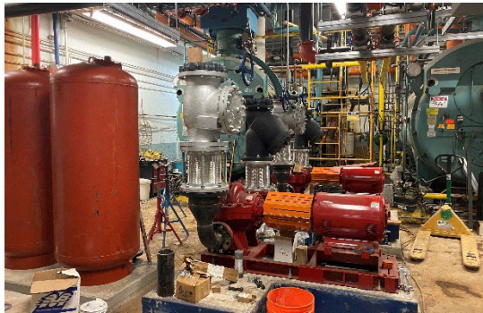
GP South Mechanical Equipment Install
