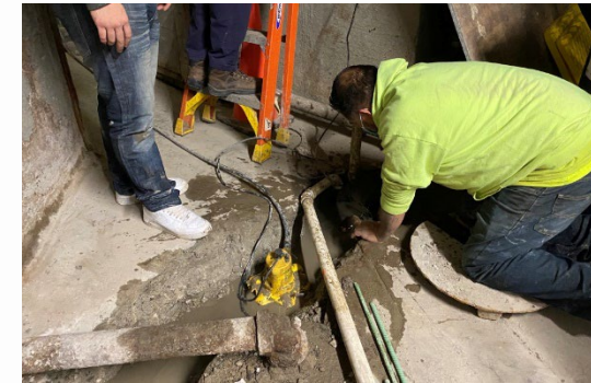
GP South Tunnel Repairs
