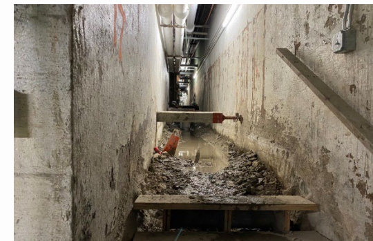
GP South Tunnel Repairs
